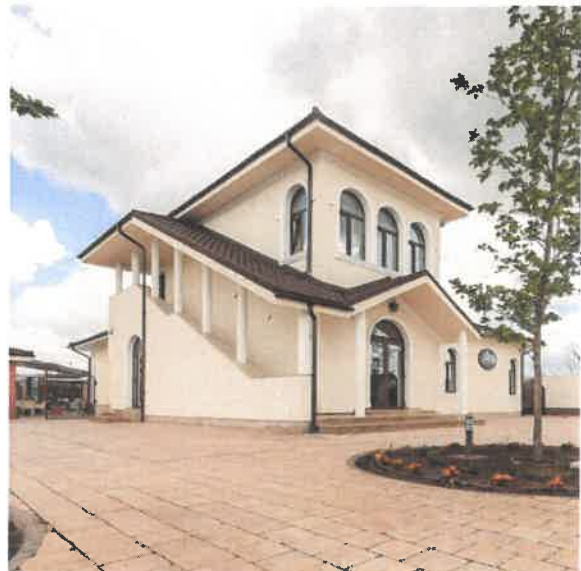
Restaurant La Conac, Balotești
